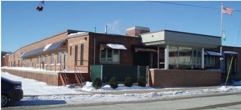
Figure G-50. VRF-2 Exterior
