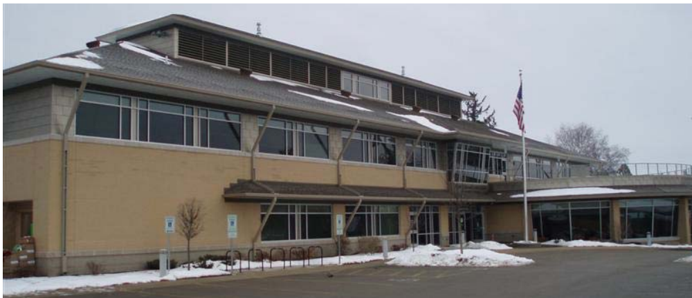
Figure G-40. VRF-1 Exterior
