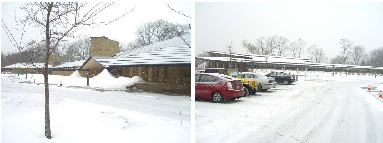
Figure G-35. Left: RAD-3 Exterior A & B Wings. Right: RAD-3 Exterior C & D Wings
