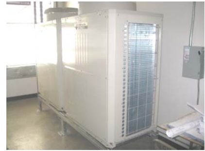
Figure G-62. VRF-3 Heat Recovery Unit
