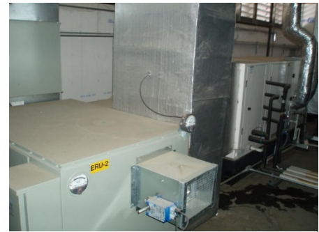
Figure G-41. VRF-1 Rooftop Unit With ERU
