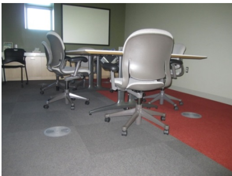
Figure G-11. DV-2 Supply Diffusers
