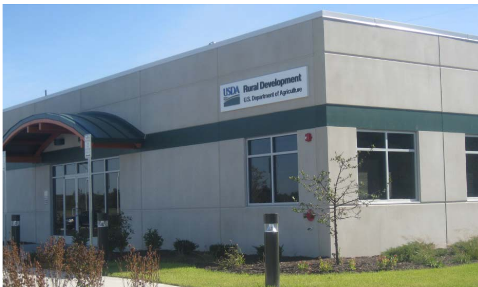
Figure G-59. VRF-3 Exterior
