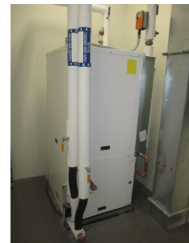
Figure G-11. DV-2 Heat Pump
