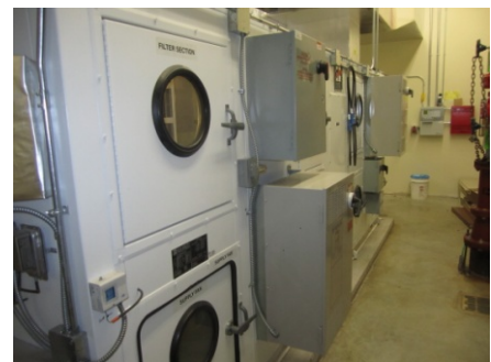
Figure G-2. DV-1 AHU-1 (100% OA)
